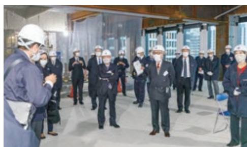
Tour of a construction site (Yokohama Gate Tower Project)
