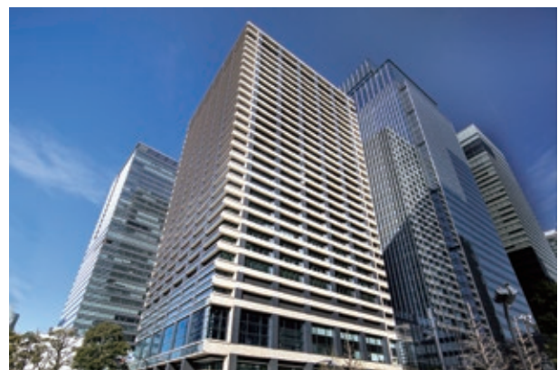
(Above) Images of digital twin (left: virtual building; right: actual building) (Below) Otemachi One
