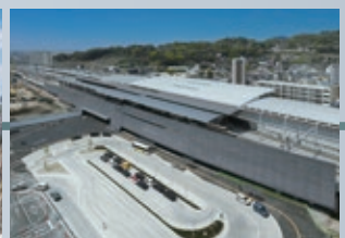
Kyushu Railway Company Kumamoto Station Building, Addition of Floors
