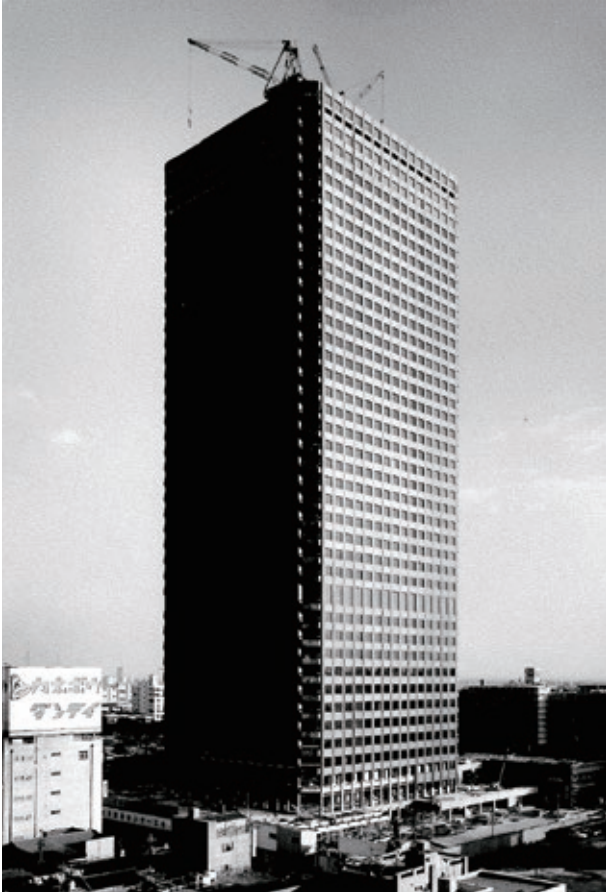
World Trade Center Building under construction in 1969 (Minato-ku, Tokyo)
