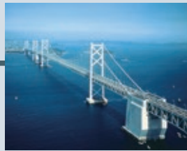
Honshu-Shikoku Bridge Project
