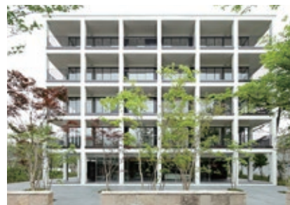
Building using precast concrete panels
